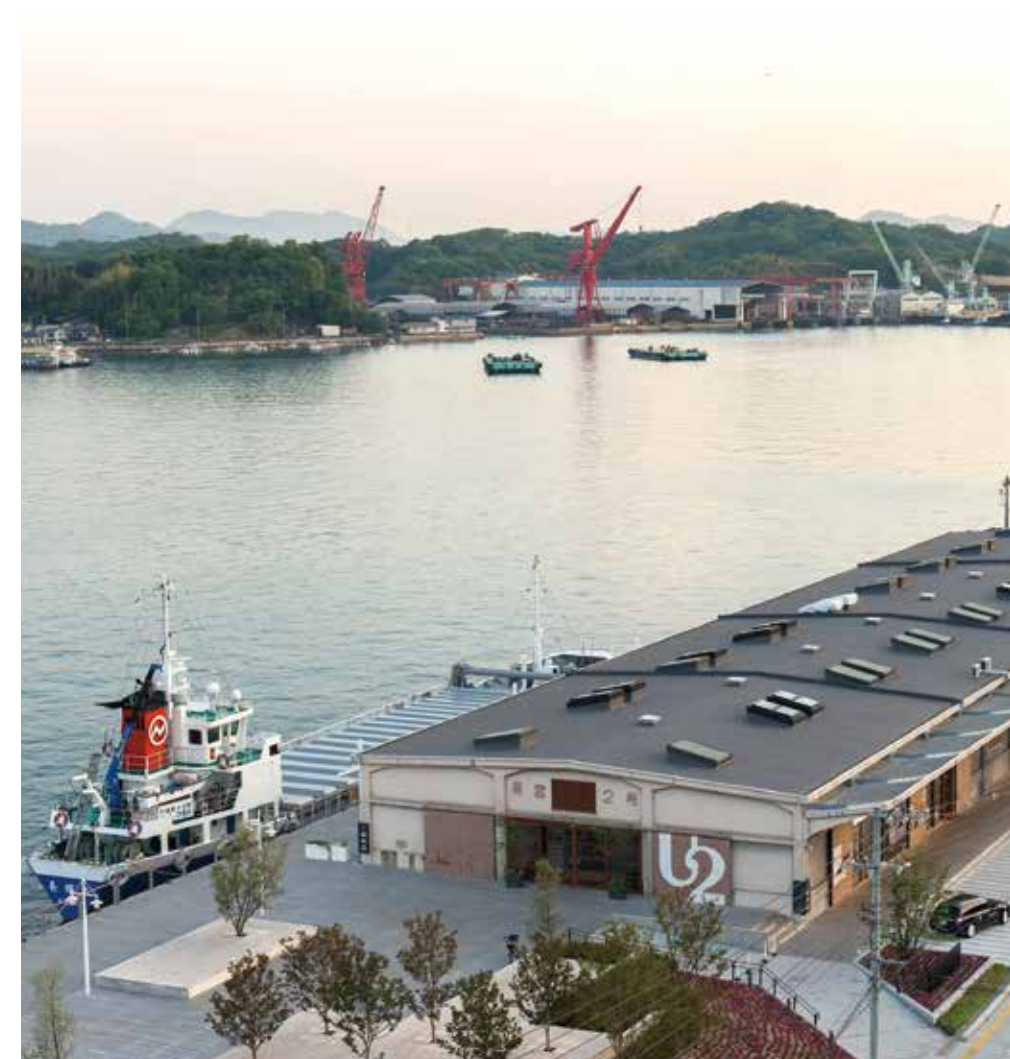
Architect: Tanijiri Makoto · Ai Yoshida | SUPPOSE DESIGN OFFICE
