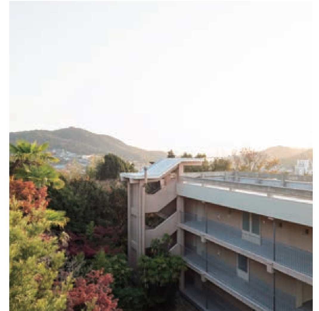
Architect: Bijoy Jain | STUDIO MUMBAI ARCHITECTS
