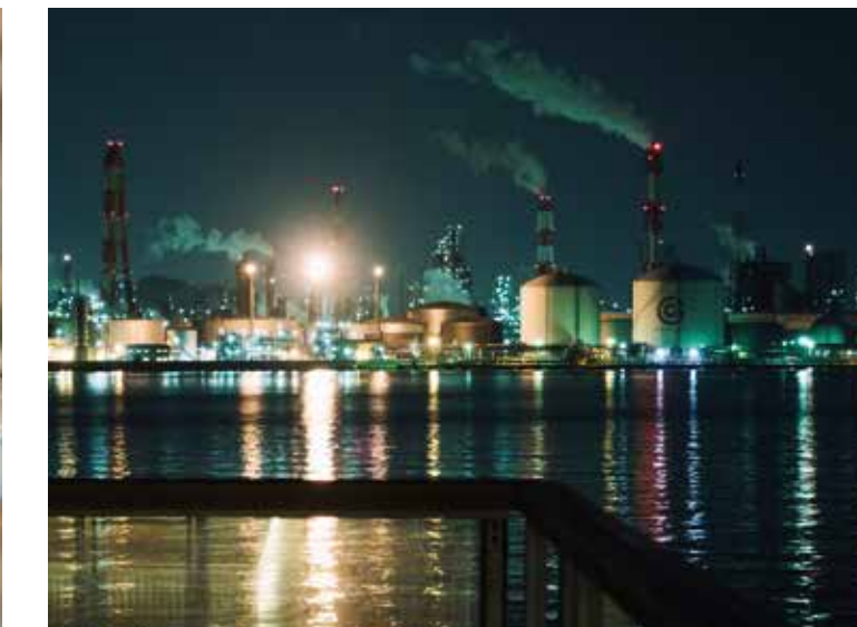
Night view of the Mizushima Industrial Complex
